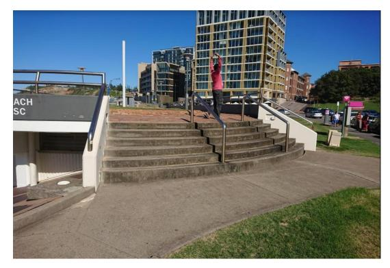
Consistent pattern at city coastal infrastructure. Similar arrangement at Parnell Place park. Note balustrades provide additional handrails to the flanks. Could still accommodate flanking bleachers.
