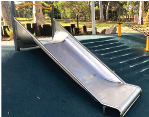
1.5m high by 1m wide embankment slide
