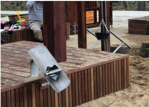
Sand Channel with membrane wheel
