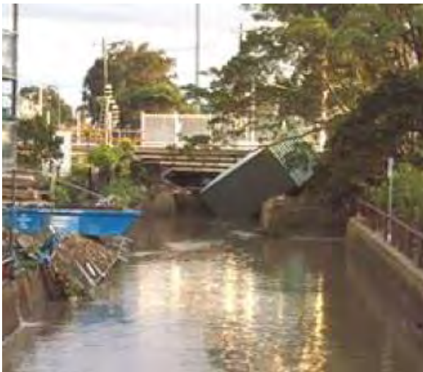
Figure 6-3. Structure blockage near outlet of Cottage Creek (Source: BMT WBM, 2008a)
