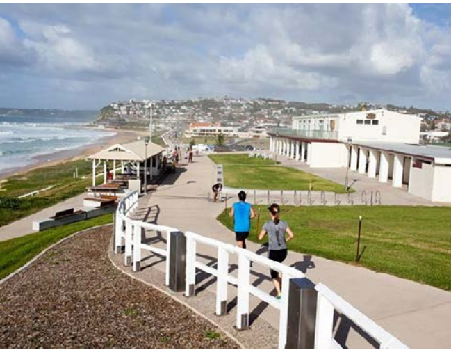
Fencing along the Newcastle Bathers way coastal walk, made from recycled wood and plastic materials
